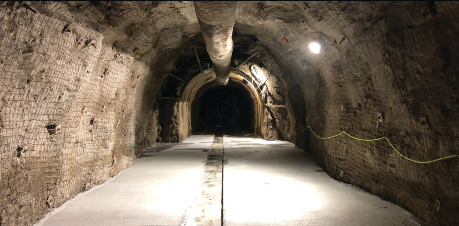
▲ To rescue the stranded TBM, Affholder constructed a recovery shaft and tunneled back toward the machine.
