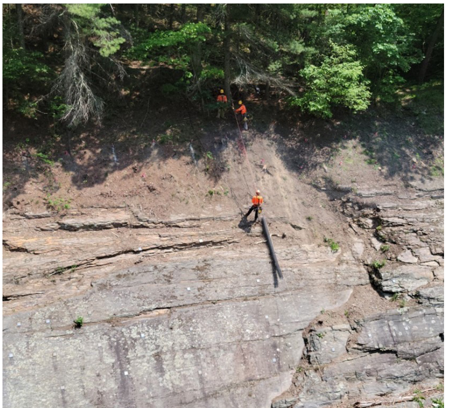
Figure 9, Placement of pinned Geobrugg Tecco® mesh
