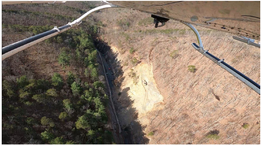
Figure 10, Aerial view of temporary access path installation during helicopter material deliveries
