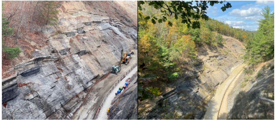
Figure 12, Finished shear blocks, one week following initial staining in November 2022 (left) and after 11 months of weathering/patina (right)
