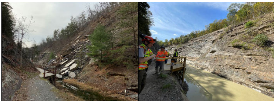
Figure 17, Paw Paw Slope Stabilization Project – As viewed looking south at the 2016 rockslide (November 2020 on left and October 2023 on right)
