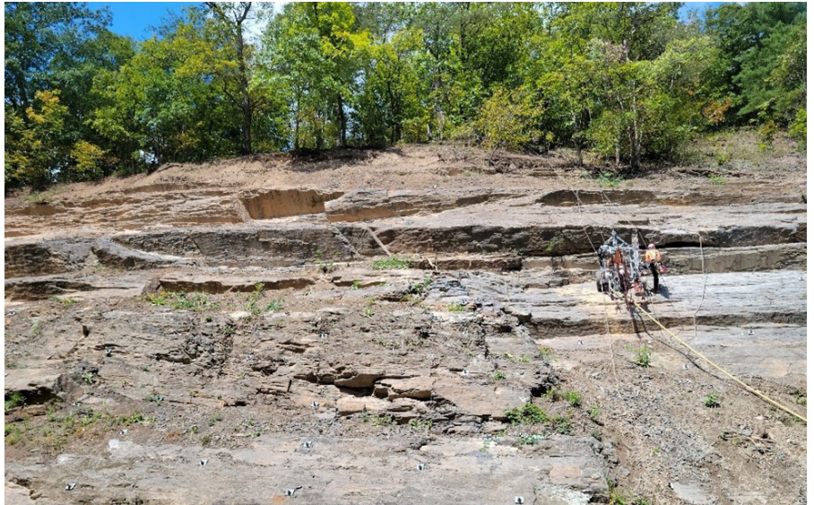
Figure 8, Rock anchor installation by rope access and wagon drill, typical
