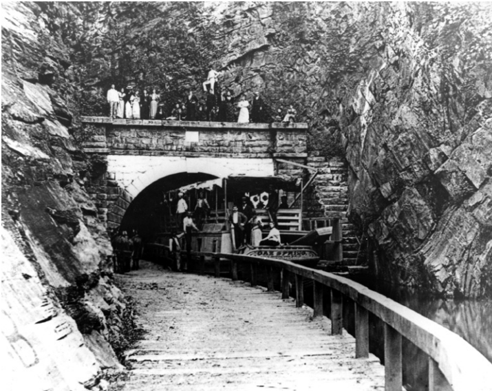
Figure 2, Paw Paw Tunnel and North Approach through the Deep Cut, 1890
