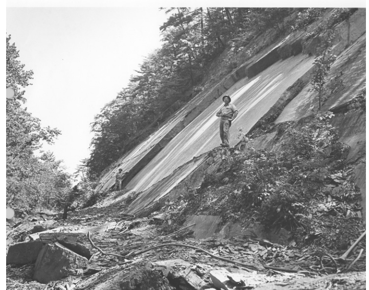
Figure 3, Rock bolting and scaling by NPS in 1950s
